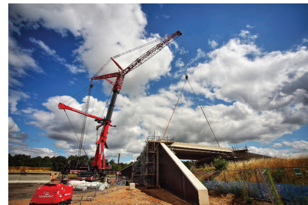
Above: Lifting in new bridge beams above the East Coast Main Line as part of the Great Yorkshire Way scheme. This £56m project was funded through the SCRIF programme with support from the private sector and Local Authority resources. The new link to the M18 motorway achieves multiple objectives through an integrated solution; improving connectivity to Doncaster Sheffield Airport, enabling access to housing and commercial employment sites, and unlocking the logistics hub at Doncaster iPort. Image courtesy of Doncaster Metropolitan Borough Council.
